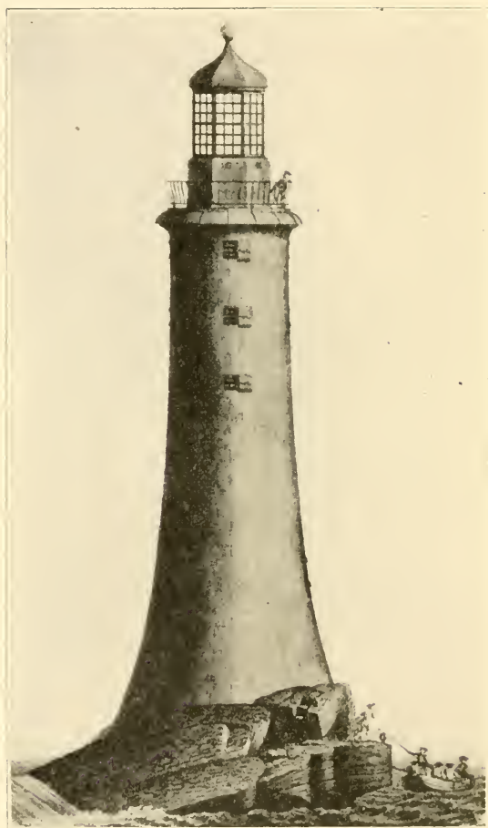
The Edystone Lighthouse, built in 1756 by John Smeaton, a noted British engineer. Repeated failures of this structure, due to lack of an efficient binding material for the stone masonry, paved the way for the invention of portland cement.
