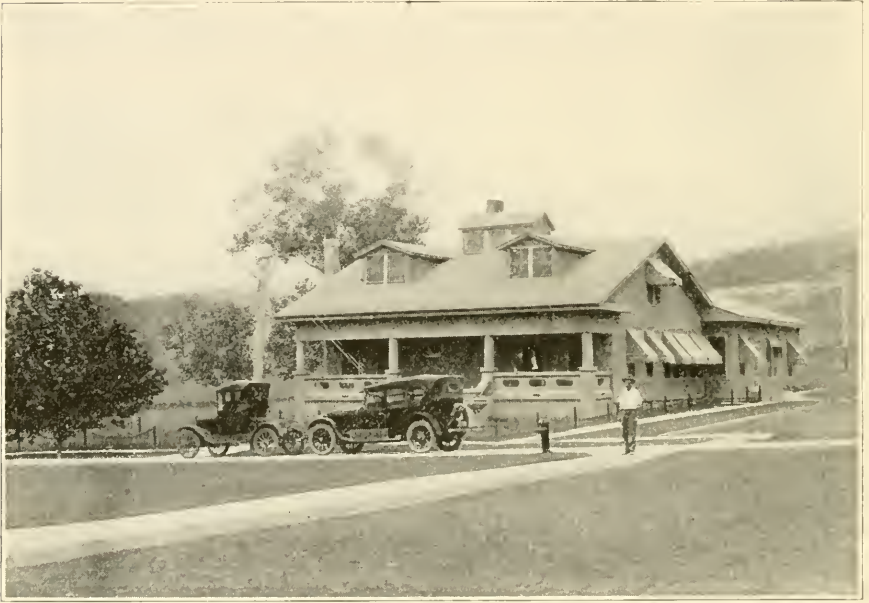
A fine example of concrete building construction in cement plant office and laboratory.
