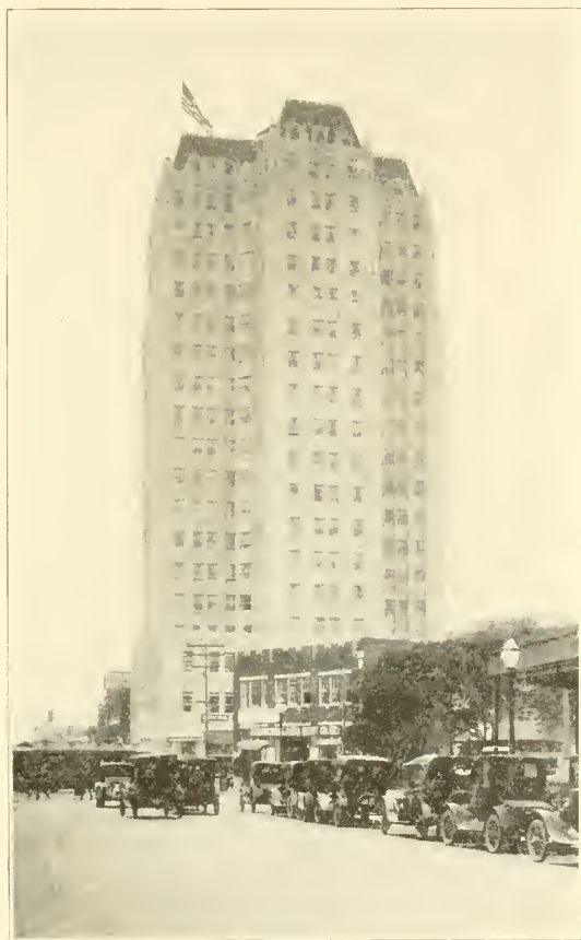
The nineteen-story Medical Arts Building, Dallas, Texas, is now the tallest reinforced concrete building in the world.
