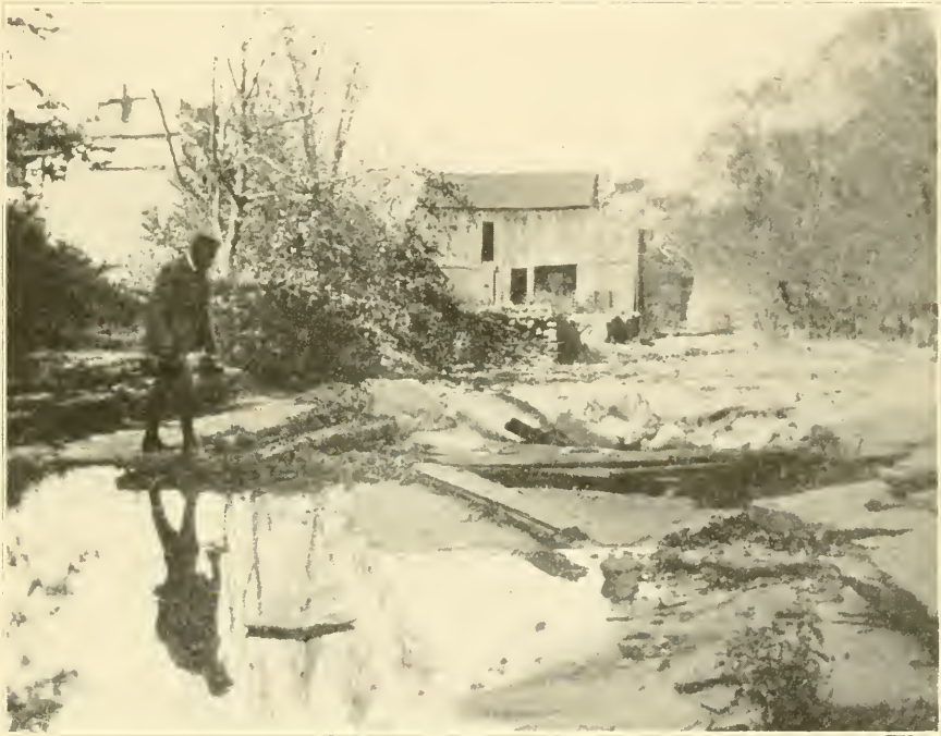
This mill at Williamsville, New York, built in 1824, supplied natural cement for the construction of the original locks on the Erie Canal at Lockport, New York.
