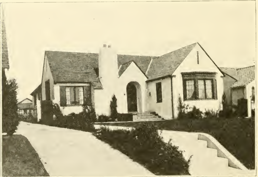
A cozy home of concrete and portland cement stucco at Hollywood, California.
