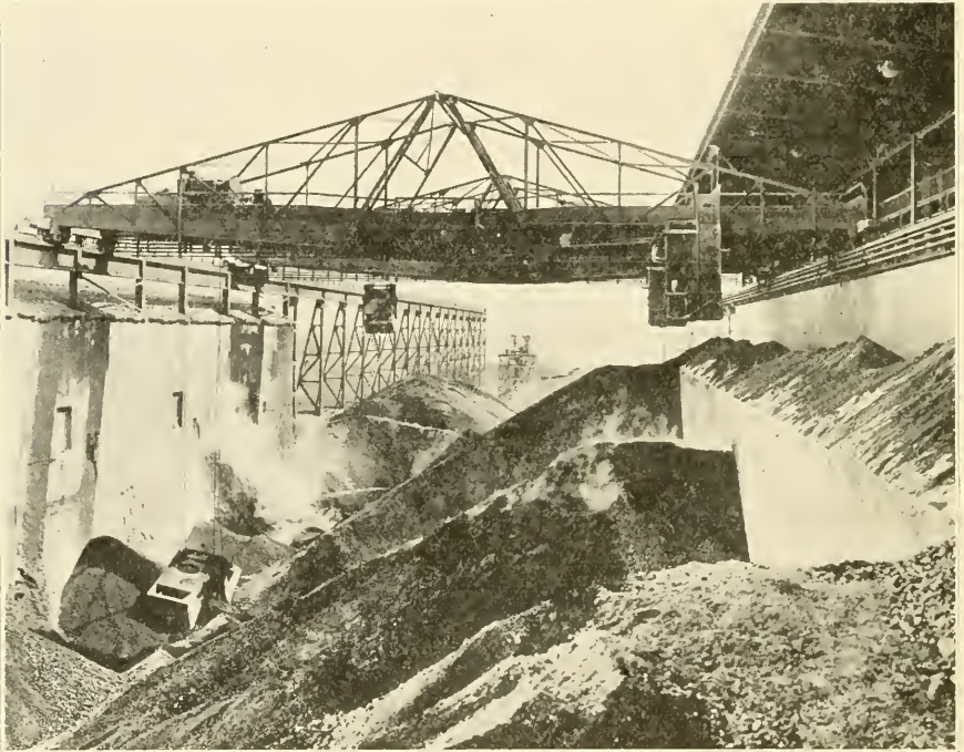
Great piles of clinker are held in reserve at most cement plants. Being impervious to the elements, it is stored until needed. Then it is ground, gypsum added, and sacked.
