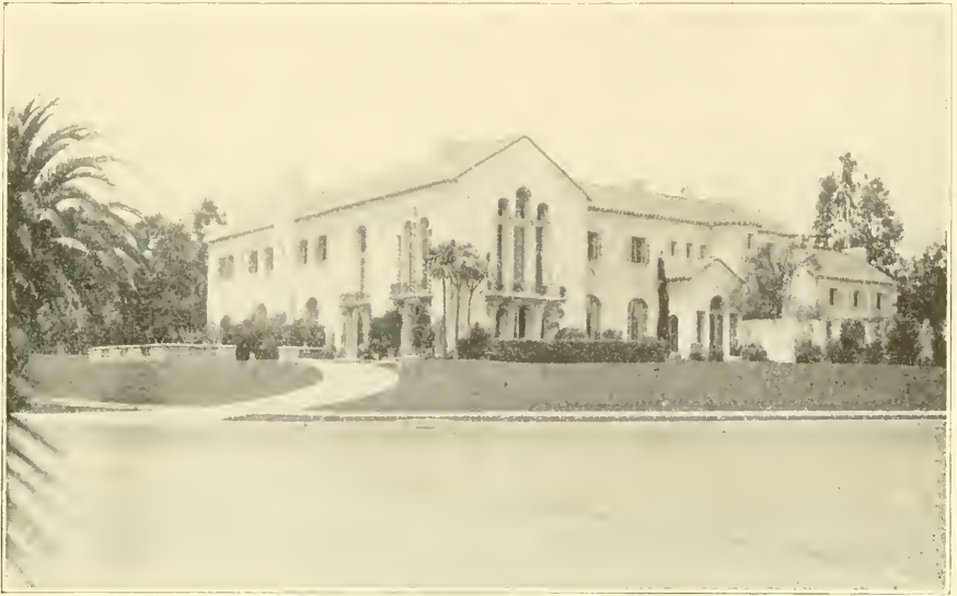
A beautiful example of portland cement stucco over concrete, at Los Angeles.
