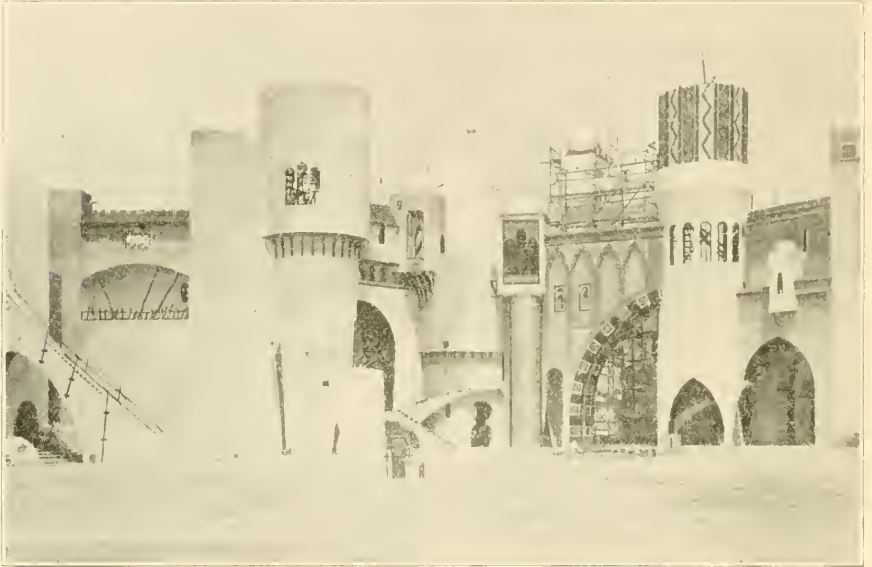
This dream city is a portion of the setting and courtyard for Douglas Fairbanks' photoplay, "The Thief of Bagdad." Both the courtyard and the buildings are of concrete.
