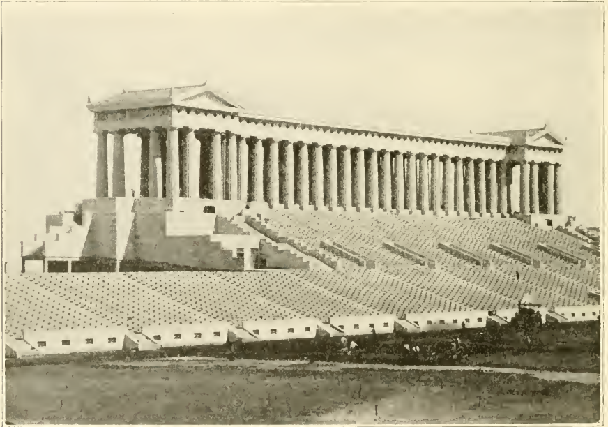
The east side of the Grant Park Municipal Stadium on the Lake front at Chicago is built entirely of concrete and faced with precast concrete stone. When the Stadium is completed, more than 100,000 people can be seated at one time.
