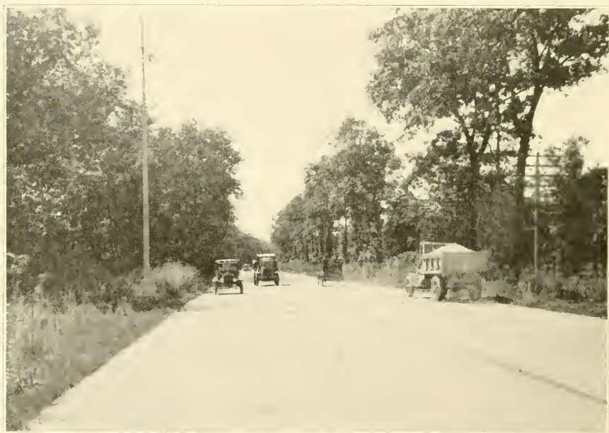
Concrete was used in the construction of the forty-foot wide "Ideal Section" of the Lincoln Highway.
