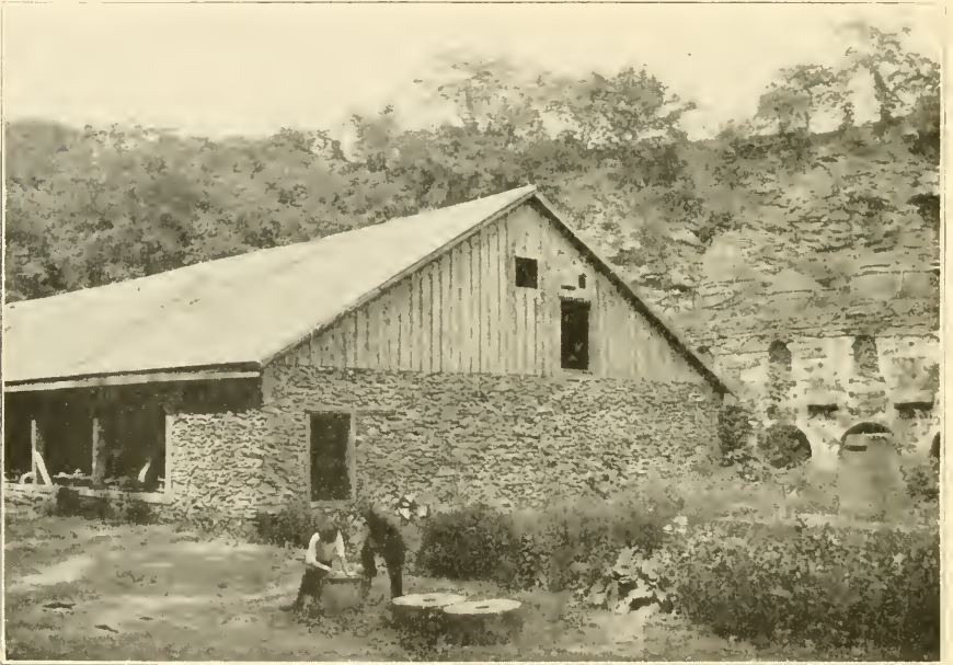
In the early days, cement was stored in bins in this and similar buildings until it was shipped to the consumer in barrels.
