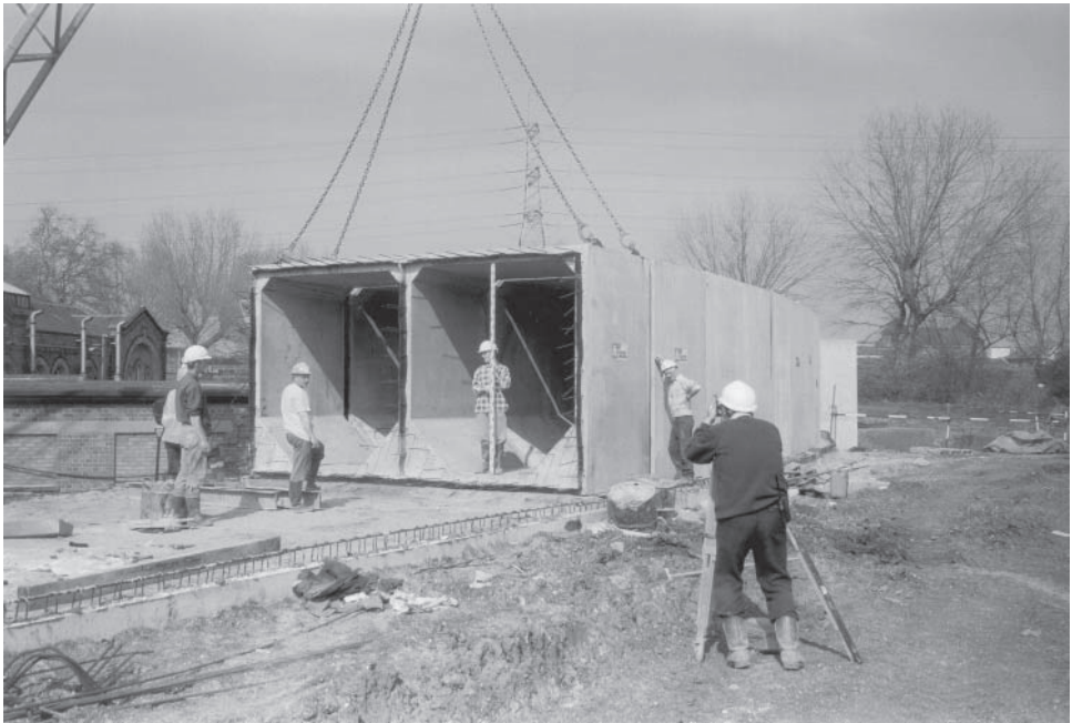
Figure 21.8 Setting one of a batch of precast culvert elements onto a prepared foundation. Note the absence of falsework and formwork. ( Courtesy Hanson Concrete Products Ltd. )
