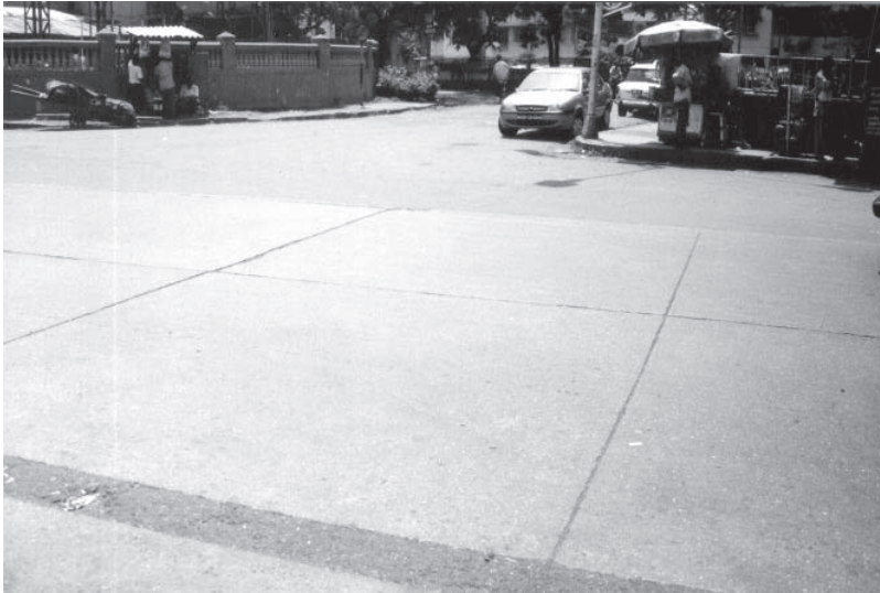
Figure 22.2 A Bombay street scene using mass concrete construction.
