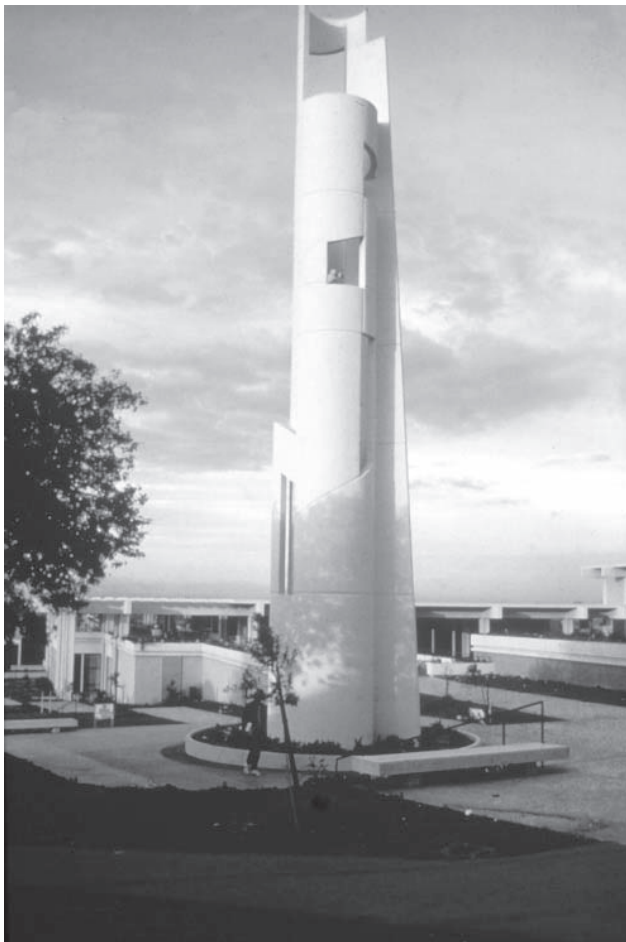
Figure 10.8 Ventilation tower on a road tunnel.
