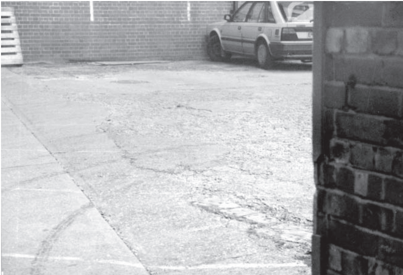
Figure 22.9 Surface abrasion.
