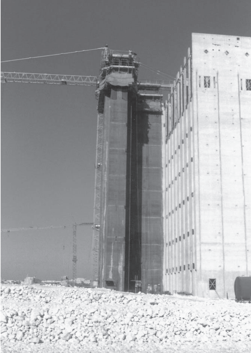
Figure 14.5 Second half of rectangular block slipformed.
