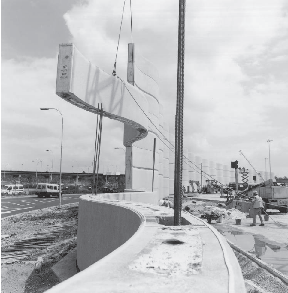
Figure 21.7 Gatwick Airport: Acoustic wall. Erection in progress, preparing to thread an element onto continuity steel, the operation to be completed by grouting after positioning the eighth tier element. (Courtesy Gatwick Airport Ltd ( BAA plc), The Pavement Team (AMECJV) and C.V. Buchan.)
