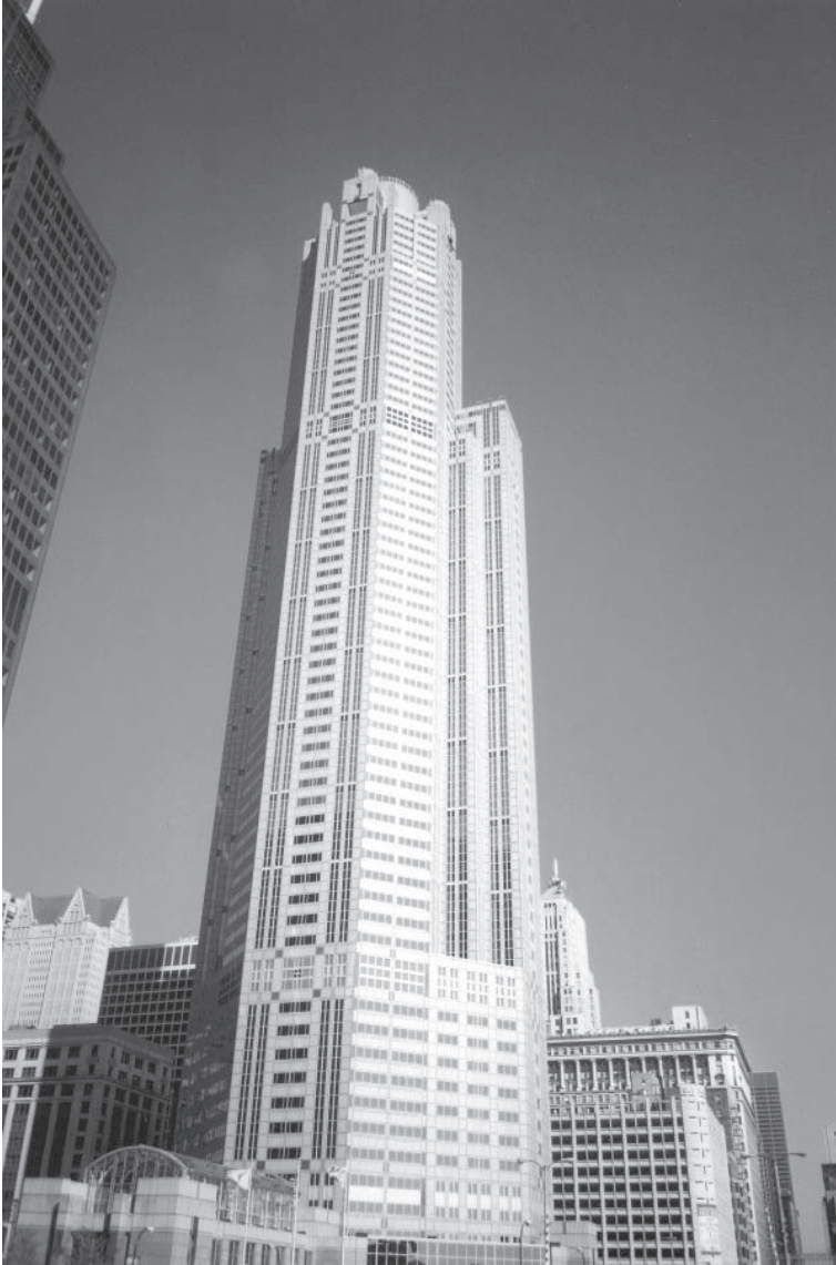
Figure 3.4 311 South Wacker Drive, Chicago – high strength concrete used in columns.
