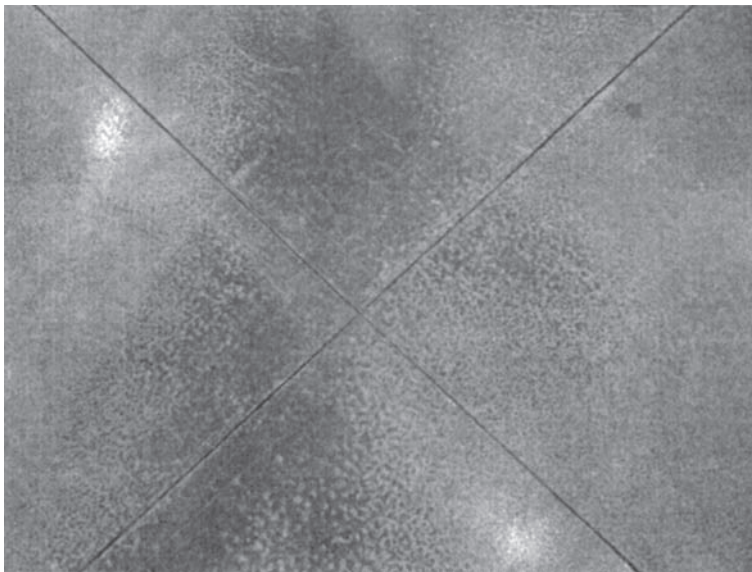
Figure 24.13 Joint strip inserted into joint immediately after curing and saw cutting.
