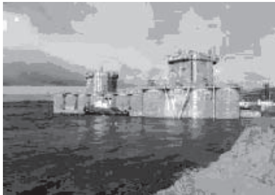
Figure 13.3 BP Harding gravity base structure used lightweight aggregate concrete with temperature limits shown in the example specification. Note that the values are much higher than normally specified. No special thermal curing procedures were necessary and there was no evidence of early thermal cracking.
