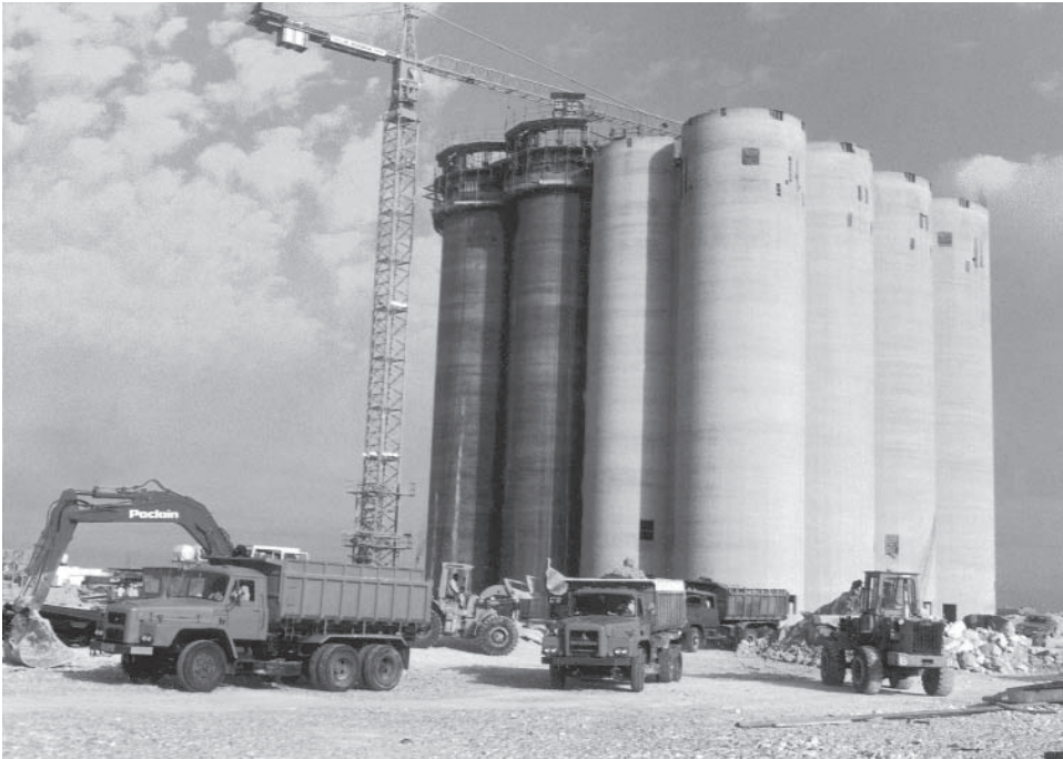
Figure 14.4 Second group of circular silos slipformed.
