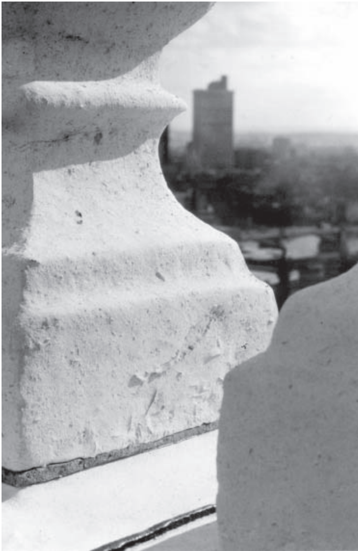
Figure 19.14 Effect of acid precipitation on Portland stone.
