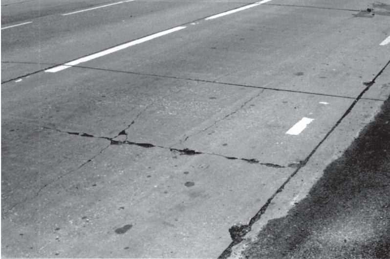
Figure 22.7 Fatigue cracking.
