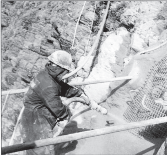
Figure 10.5 Nozzleman at work.
