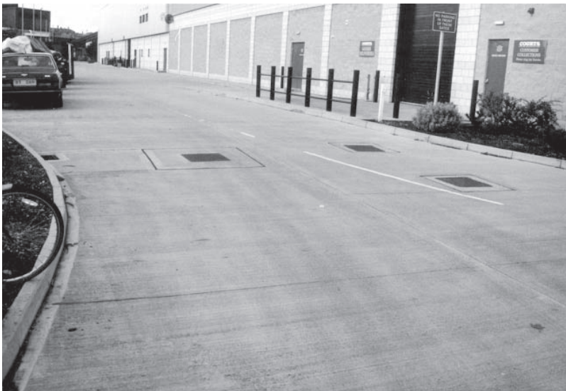
Figure 22.1 A typical industrial lorry yard.
