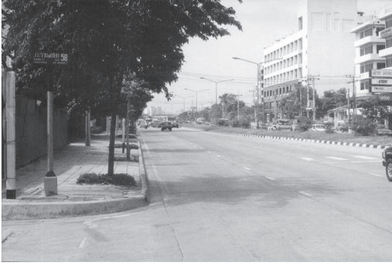
Figure 22.3 Bangkok reinforced concrete pavement.
