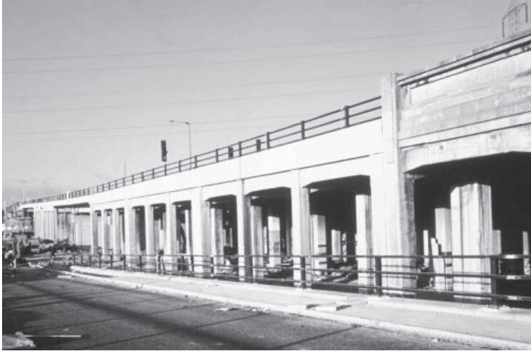
Figure 10.10 Viaduct renovation and strengthening.
