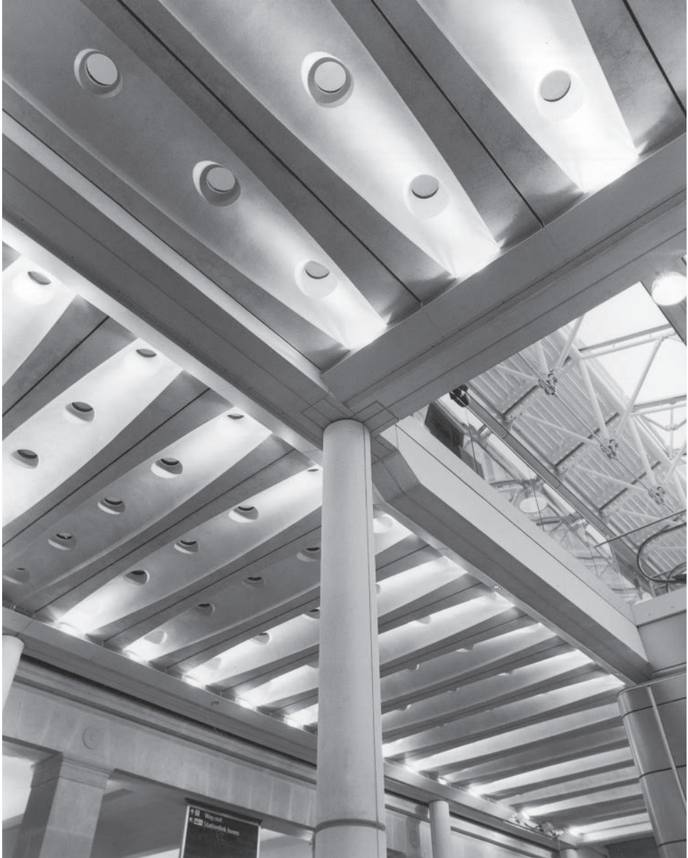
Figure 21.3 Paddington Station, London: Structural steel combined with precast and in-situ concrete, joints first bolted then welded, an elegant example of hybrid construction. (Courtesy Railtrack, Taylor Woodrow Construction and Trent Concrete Ltd.)
