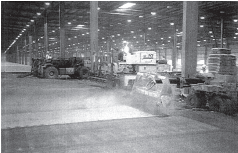
Figure 24.7 Laser screeded large area pour, using steel-fibre reinforced concrete.
