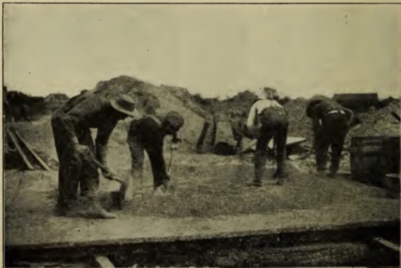
Men using square-pointed shovels turn the sand and cement thoroughly several times until the streaks of brown and gray have merged into a uniform color.
