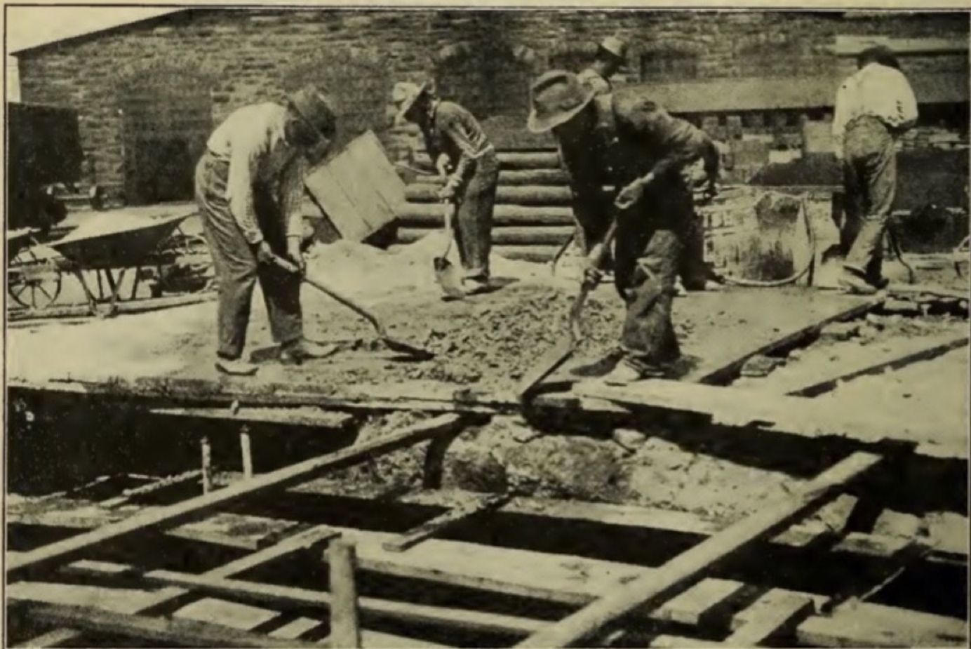
If the mixing platform can be placed near where concrete is to be deposited, the concrete may be shoveled directly from the platform into the forms.
