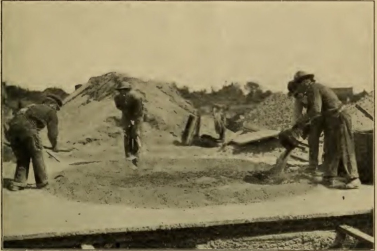
The previously wetted broken stone or pebbles are then added to the sand-cement mixture and thoroughly incorporated with it, after which a depression or hollow is shoveled in the pile and the required amount of water added.
